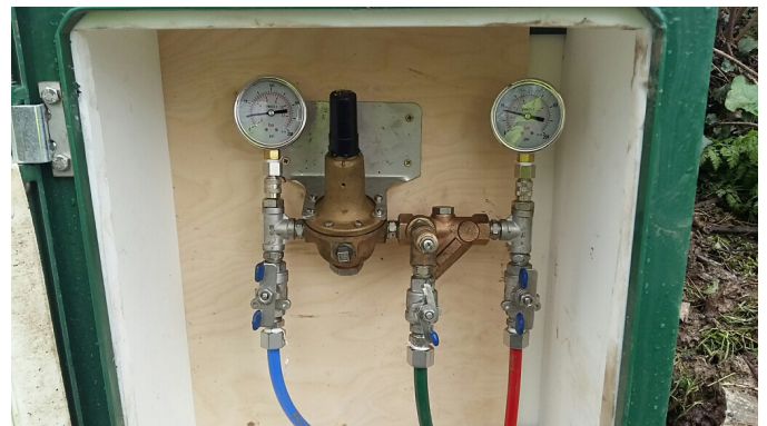
A recently installed Pressure relief valve fitted by the Find & Fix team
